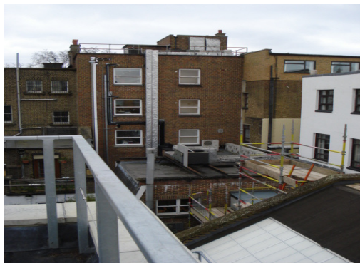
GENERAL VIEW OF ROOFSCAPE TO 184 KENNINGTON PARK ROAD AND 20 STANNARY STREET LOOKING EAST TOWARDS NUMBER 184 FROM ROOF OF 22-26 STANNARY STREET
