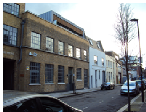
REAR ELEVATIONS TO NOS. 20 – 26 STANNARY STREET LOOKING SOUTH (INCLUDING NEW SECOND FLOOR)
