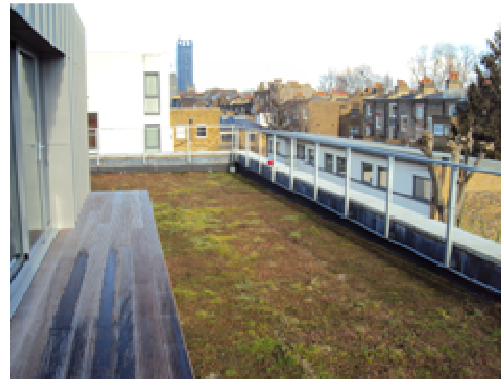
GENERAL VIEW OF ROOFSCAPE FROM NEW SECOND FLOOR SPACE LOOKING NORTH (NEW SPACE ON LEFT HAND SIDE OF PICTURE)
