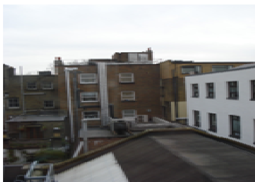
GENERAL ROOF LINE LOOKING EAST FROM NO. 20 STANNARY STREET
